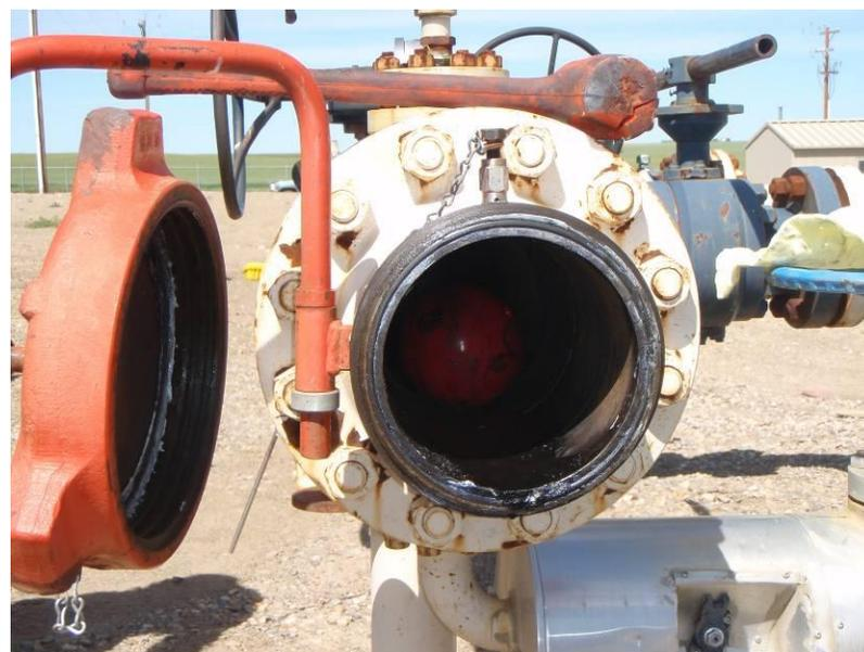
Fig. 1.3.3 – Pig Receive Trap at Crowfoot Gas Plant
