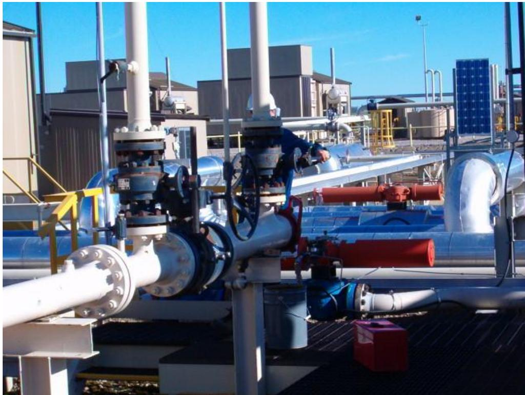
Fig. 1.3.1 - Pig Launch Facility at Severn Compressor Station
